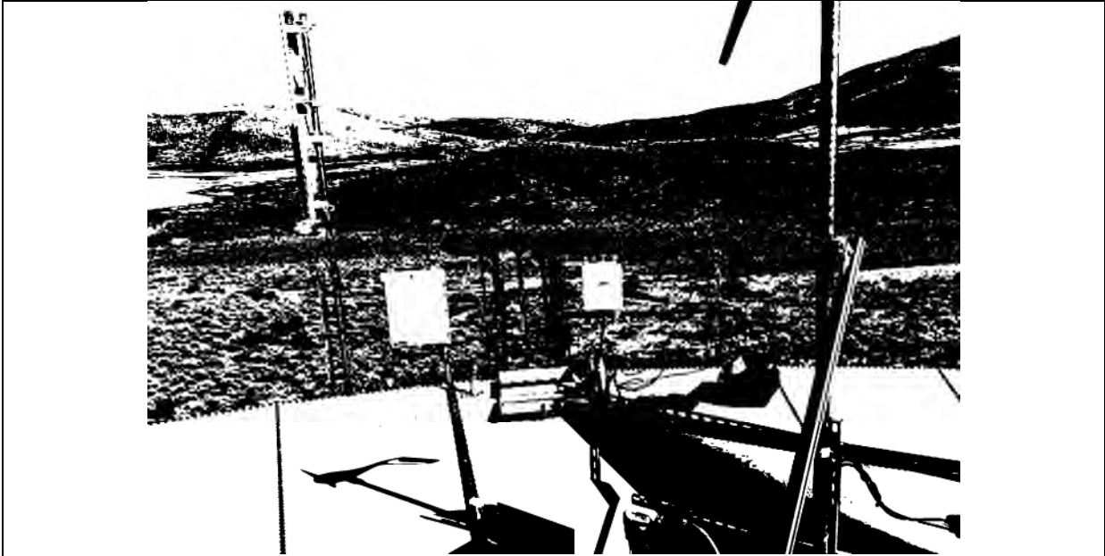
Exterior Roof railing is compliant but short
