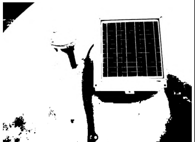
Solar panel on roof
