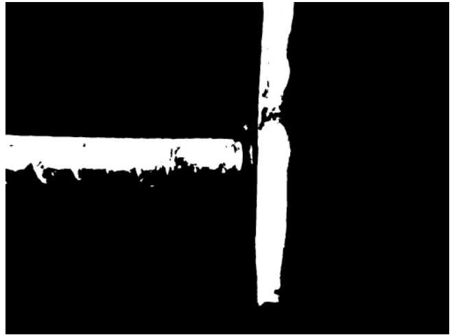
Weld on ladder
