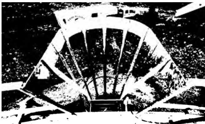
Top of safety cage
