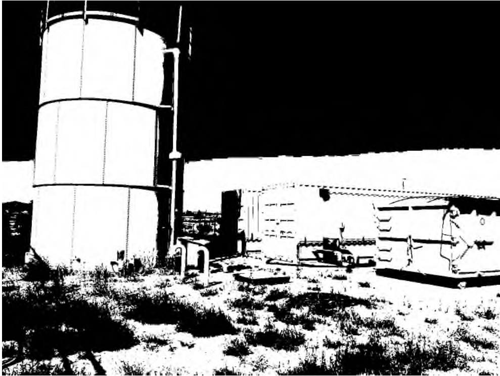
Well #11 Arsenic Treatment Backwash Tank 5
