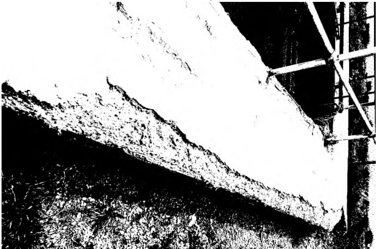
Marwood Walkway – Exposed Aggregate and Rebar
