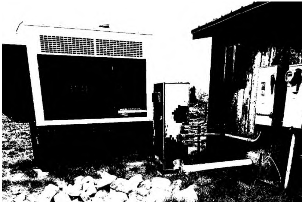
Well #10 – Exterior and Backup Generator
