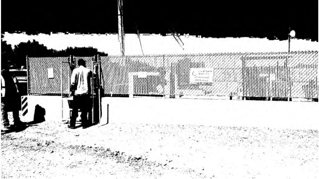
Lift Station #10 Exterior View
