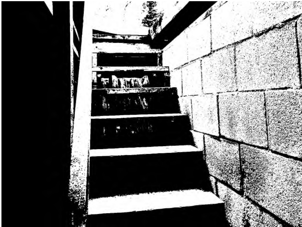
Well #14 Stairs into subarea (vault)
