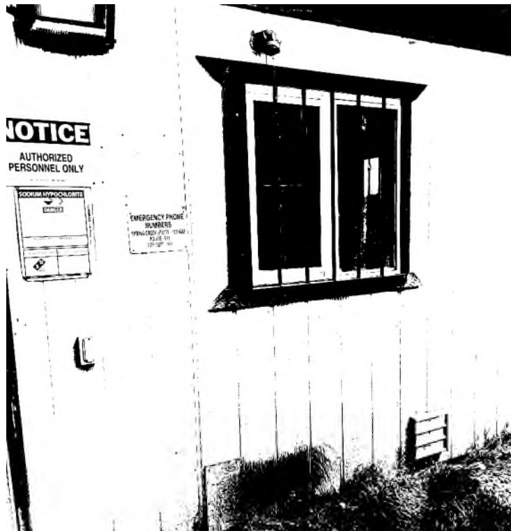
Well #7 Pump House – Outside View
