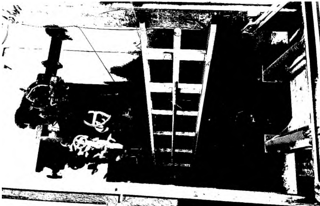
Tract 400 – Oakmont PRV (located at Oakmont and Silver Oak Drives) - Interior
