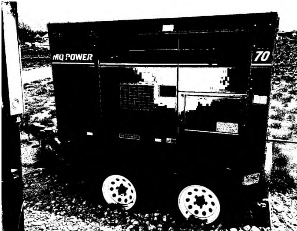
Marwood Backup Generator
