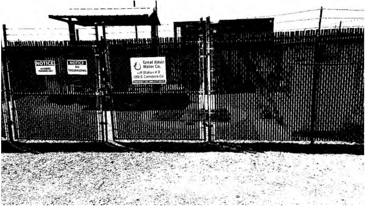
Lift Station #3 Exterior View
