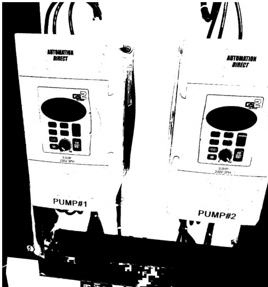
Lift Station 1 – Controls
