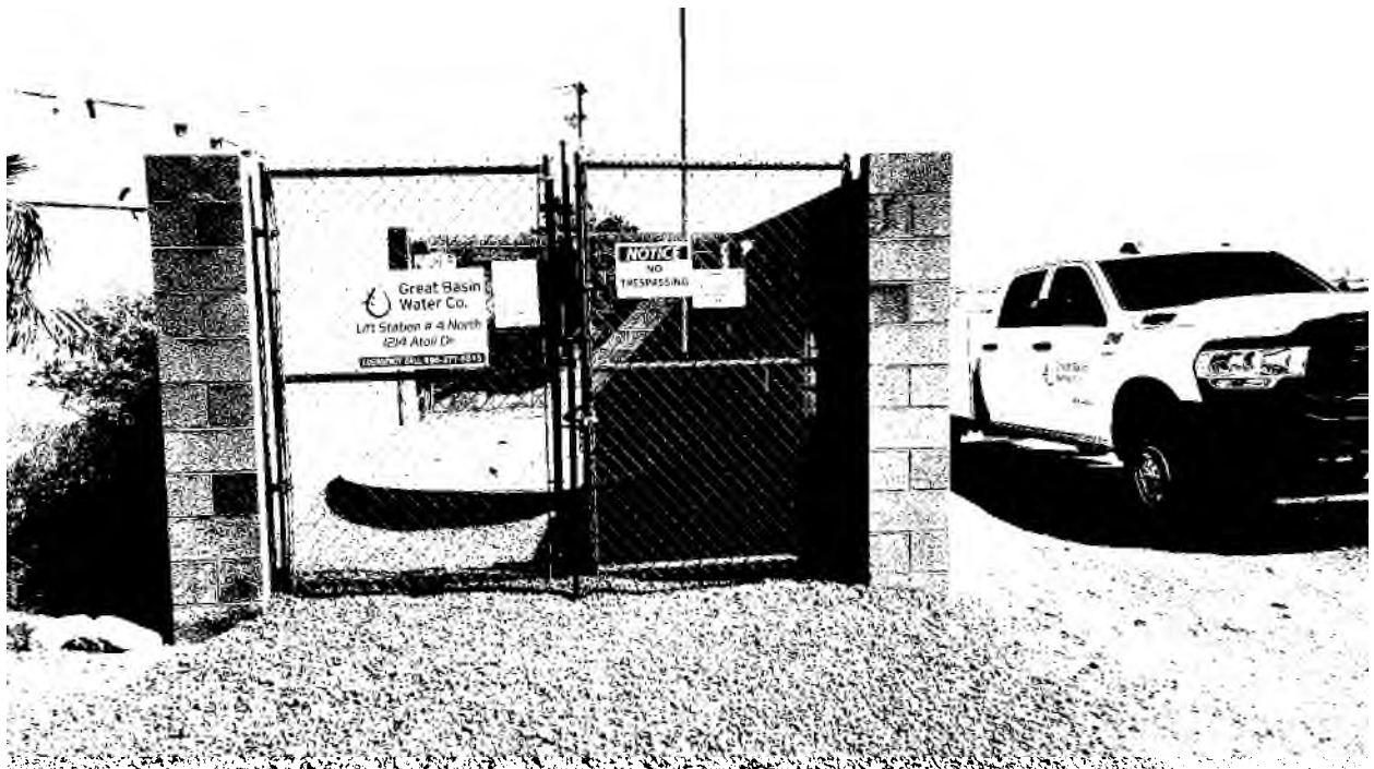
Calvada North Lift Station #4 Exterior View
