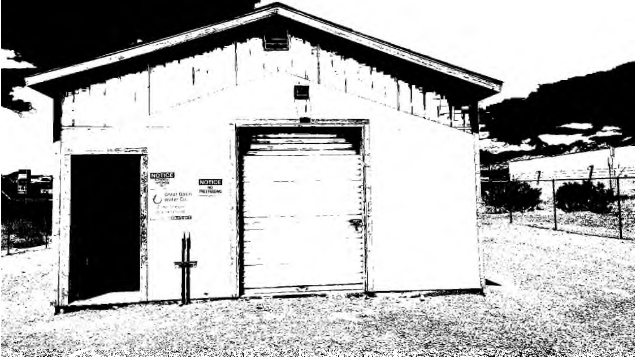
Alfa Booster Station Exterior View
