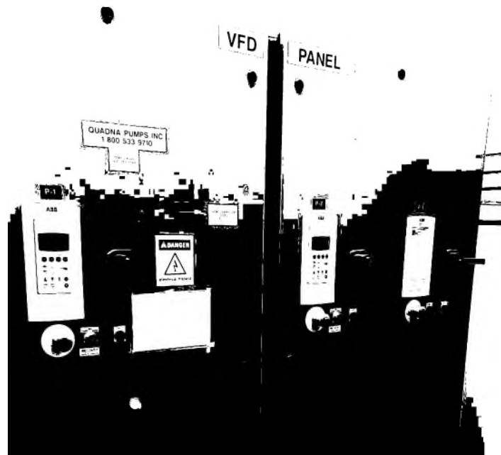
VFD Panel at Mesquite Booster Station
