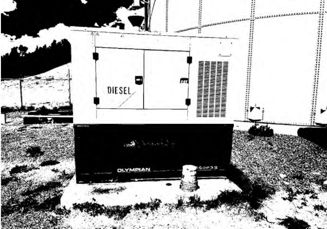
Tank 106 Site – Diesel Backup Generator Housing Tract Booster Pumps – Tract 400
