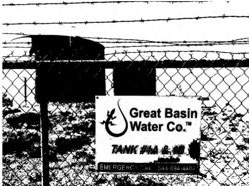
Tanks 1A and 1B
