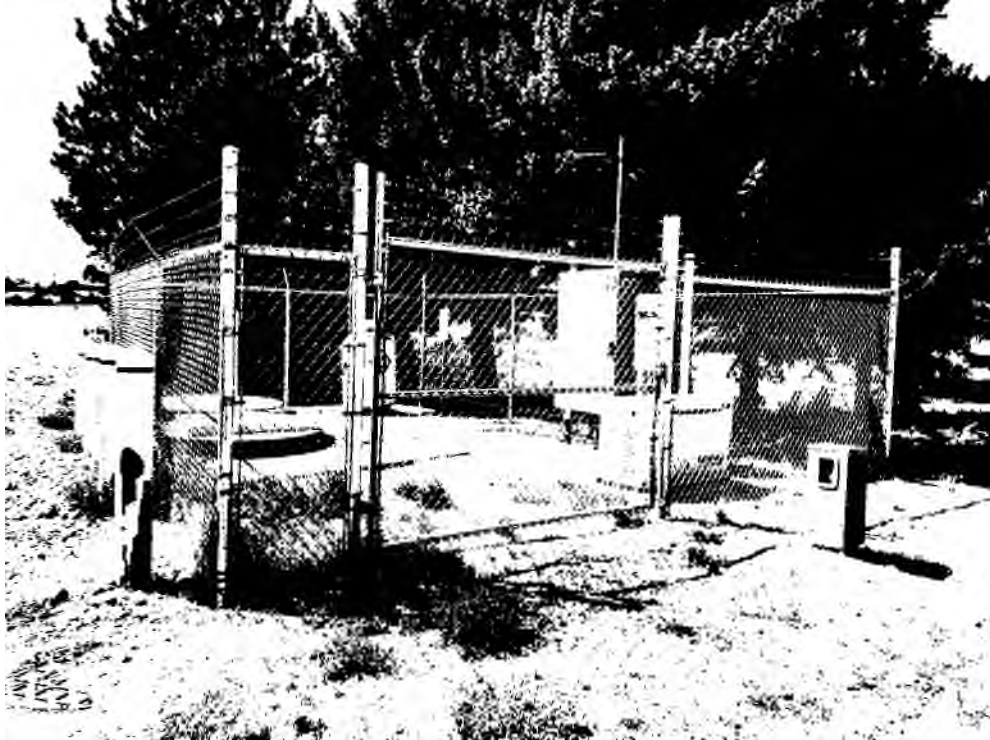
Lift Station 1 Site (Flygt Package Lift Station) 11
