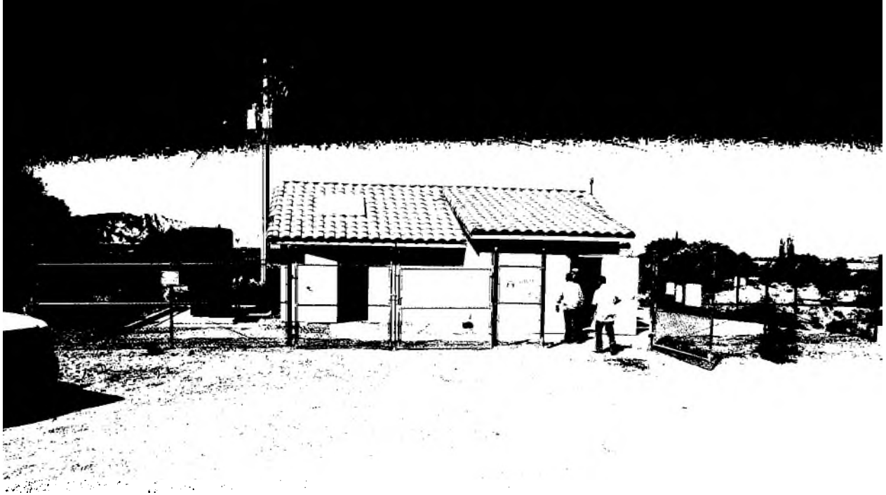
Mountain Falls Well #2 Exterior View 2
