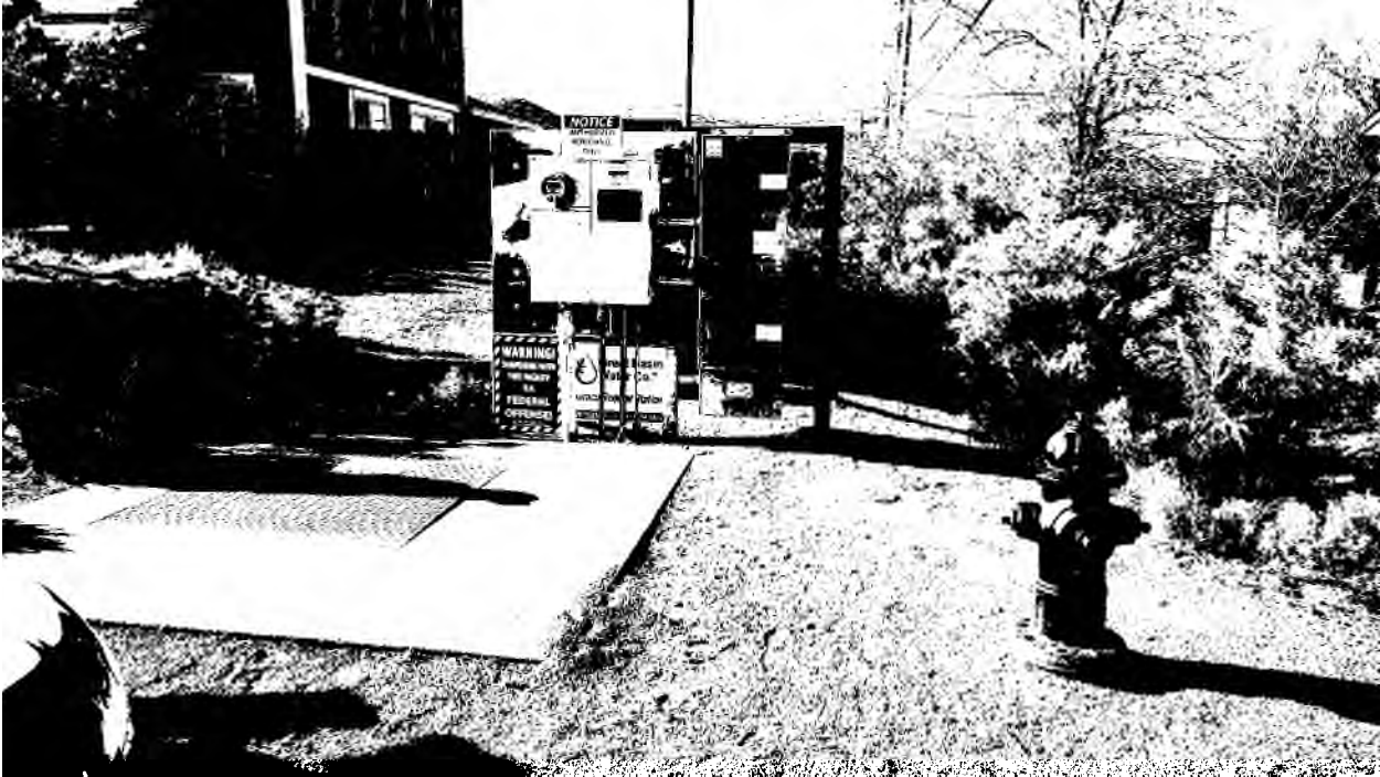
Entry to Touraco Booster Station
