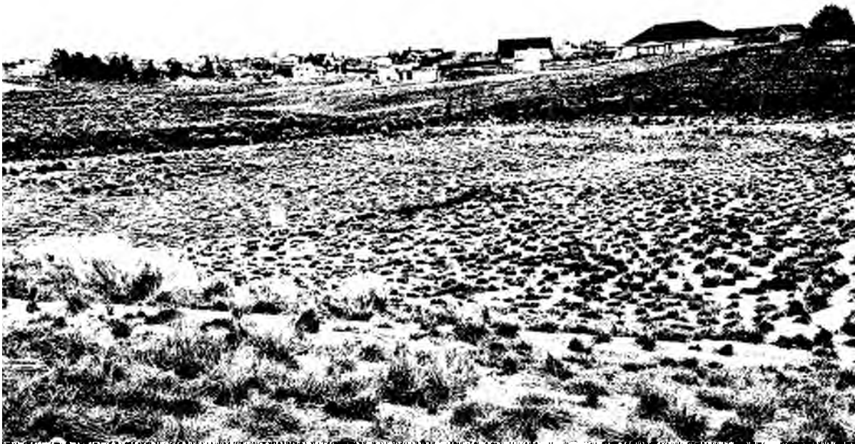
Wastewater Treatment Disposal Leach Field
