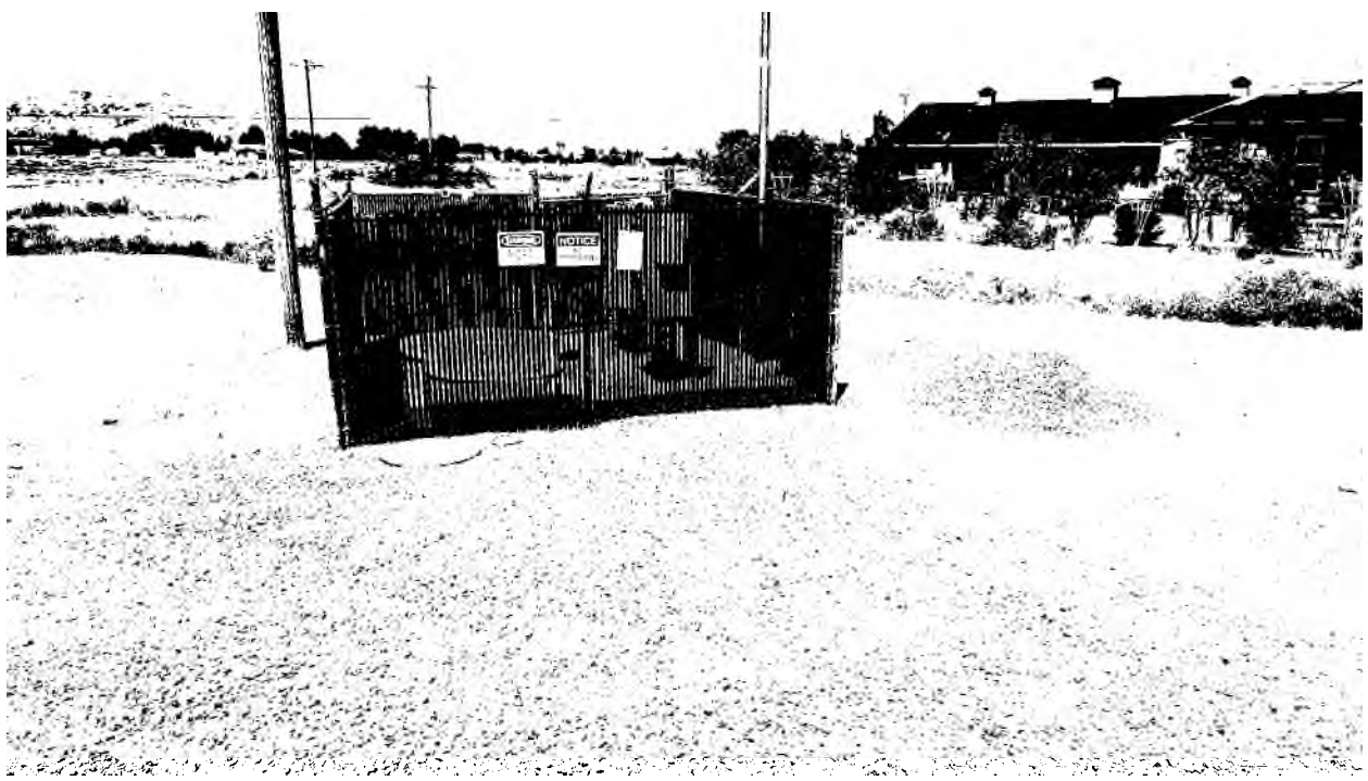
Lift Station #7 – Exterior View
