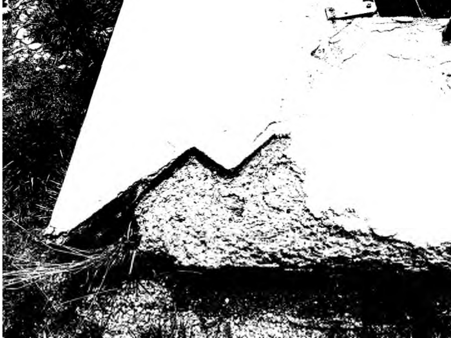
Marwood Walkway – Concrete Deterioration
