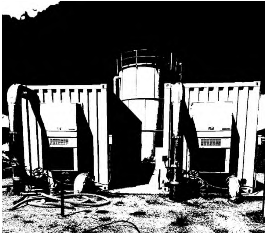
Well #11 Arsenic Treatment Twin Modules
