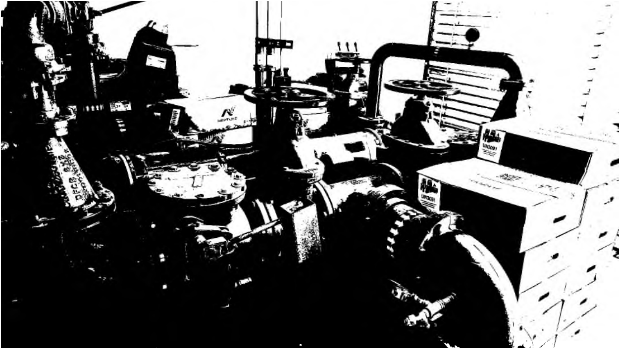
Alfa Booster Pumps #1 and #2
