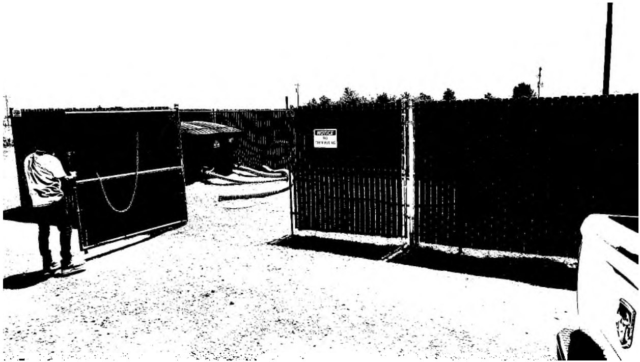
Lift Station #5 Exterior View
