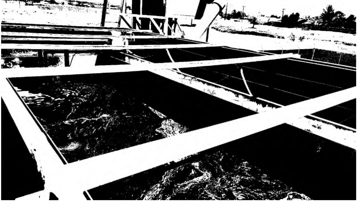
Plant 3 Sand Filter
