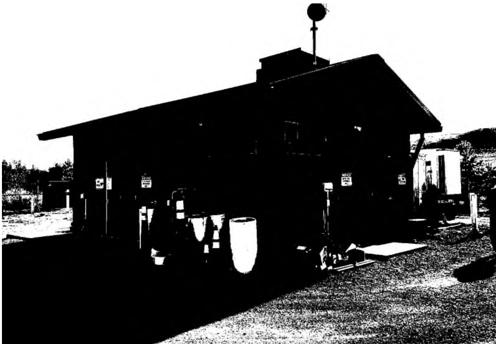
Van Dyke Well – Exterior View
