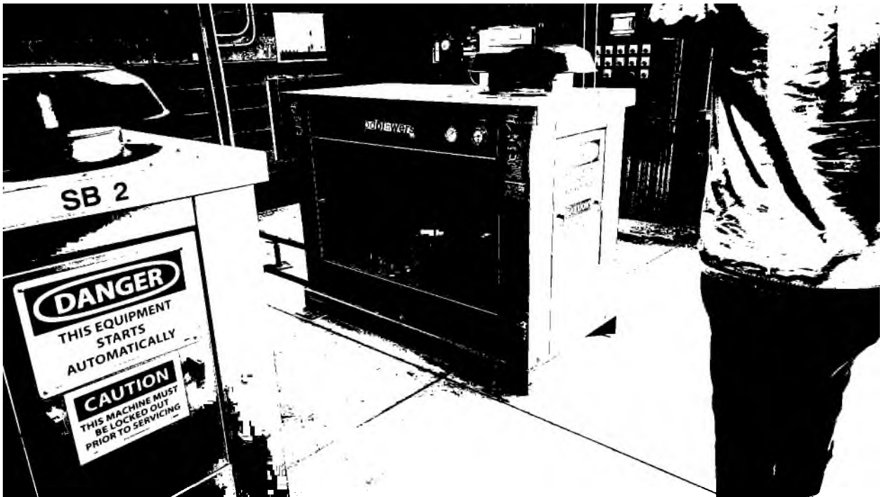
Spring Mountain Motorsports Ranch Plant Blowers
