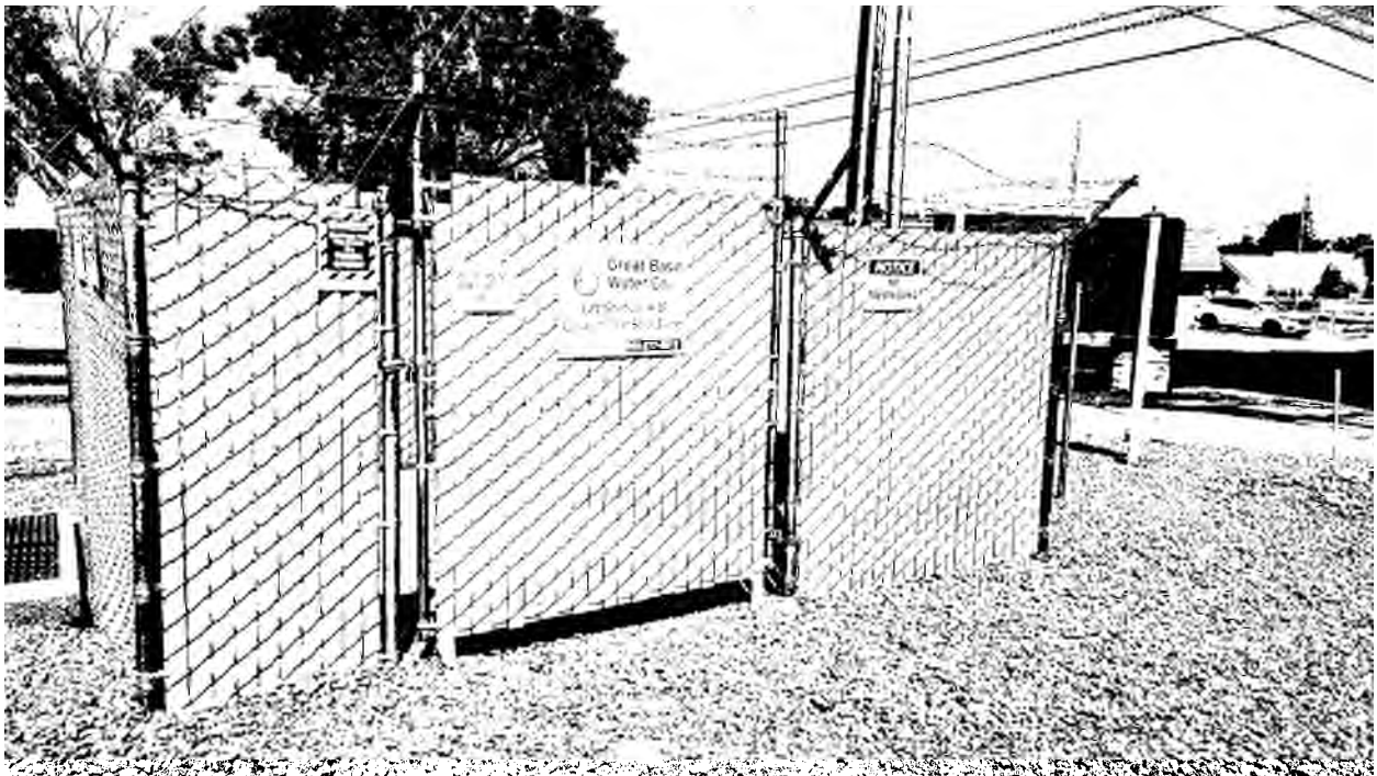
Lift Station #8 Exterior View
