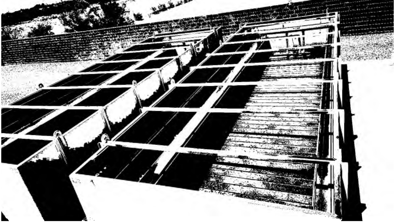
Mountain Falls Wastewater Treatment Plant Sand Filter
