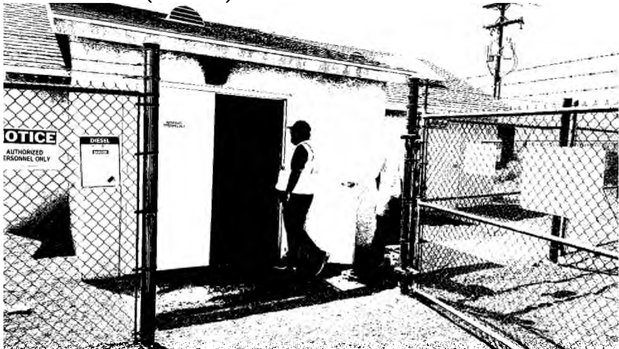
Mountain Falls Well #1 Exterior
