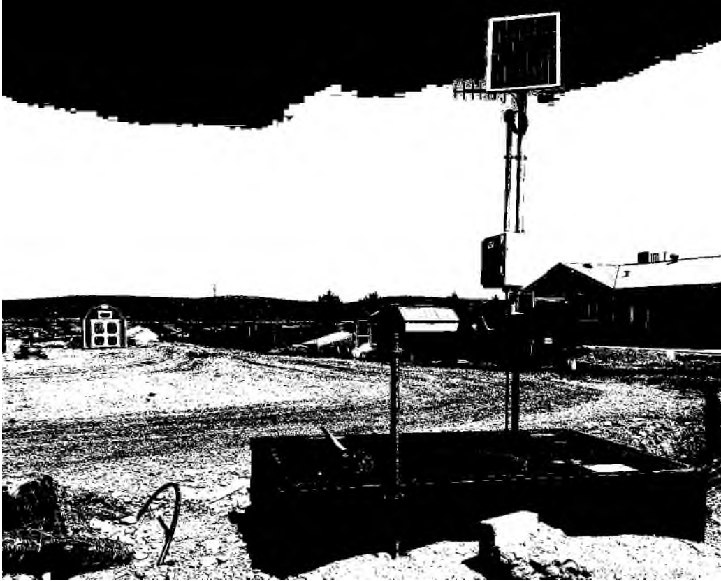
Tract 400: Wellington Pressure Reducing Valve Site – Exterior
