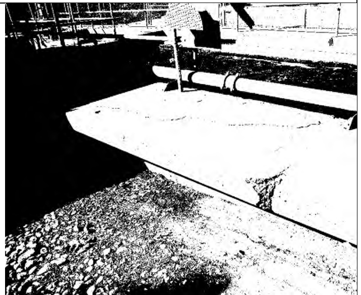
Photo 3 (9/13/2017) – Existing concrete cantilever walkway along east side of plant. Photo shows concrete cracks, spalling, and exposed aggregate.
