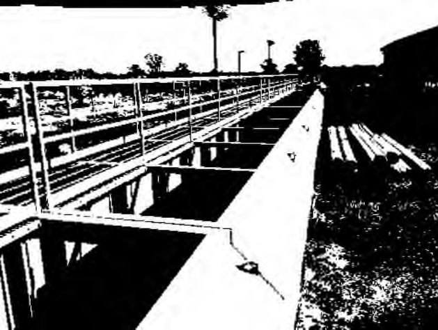
Aeration Chamber and Walkway Grates
