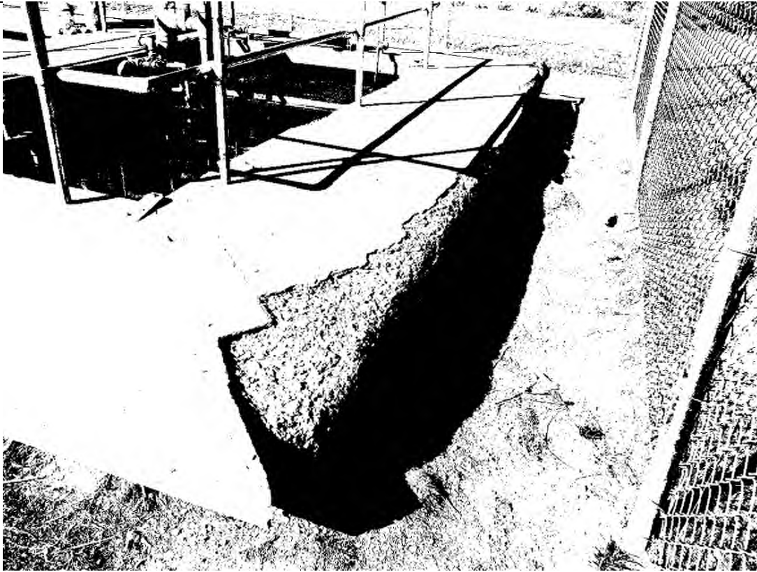
Photo 1 (9/13/2017) – Existing concrete cantilever walkway along north side of plant. Photo shows significant concrete deterioration including cracks, spalling, exposed aggregate, and exposed rebar.
