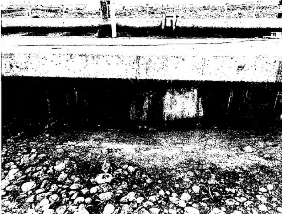
Photograph 9. Evidence of prior leakage along the east wall.
