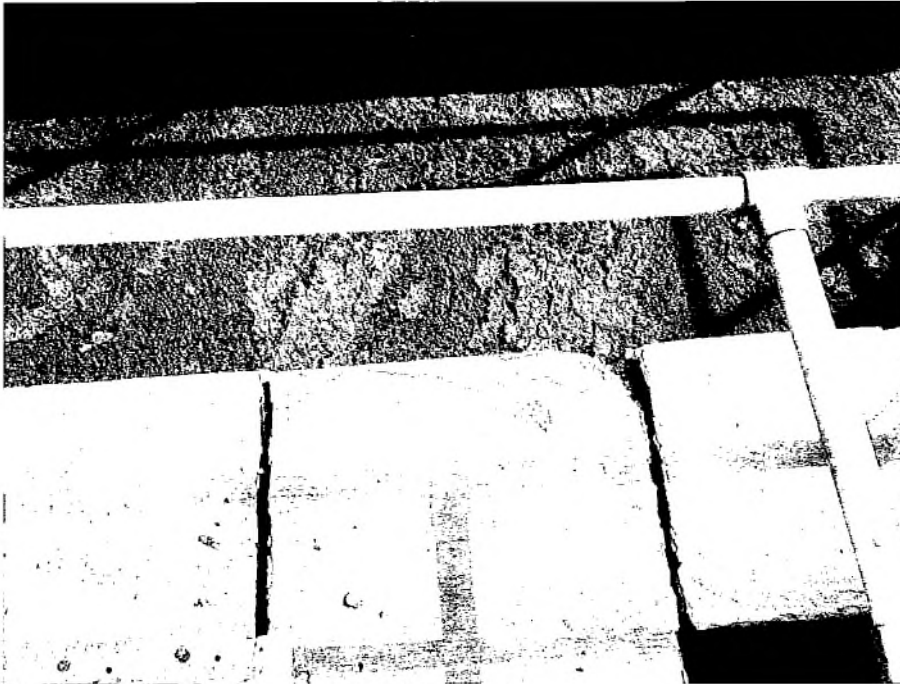
Photograph 11. Wide gaps at joints in the walkway.
