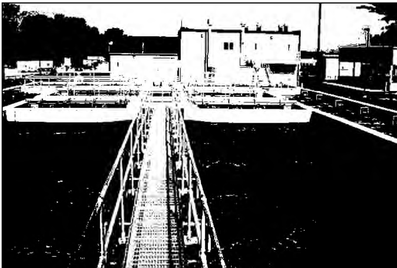
The rectangular layout of the SEQUOX Process results in a smaller footprint and easy expansion.
