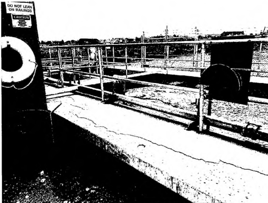
Photograph 8. Walkway overlay separating from the underlying slab.
