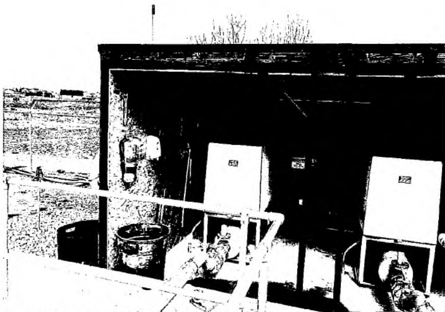
Photograph 3. Front view of the equipment enclosure.
